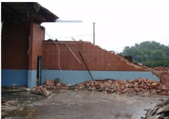
(b) After demolition
