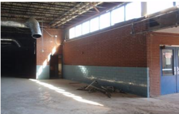
(a) Before demolition
