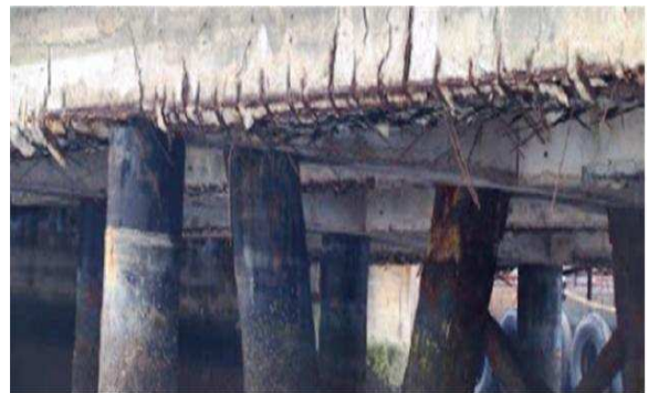
Fig. 2: View of the deck and steel piling
