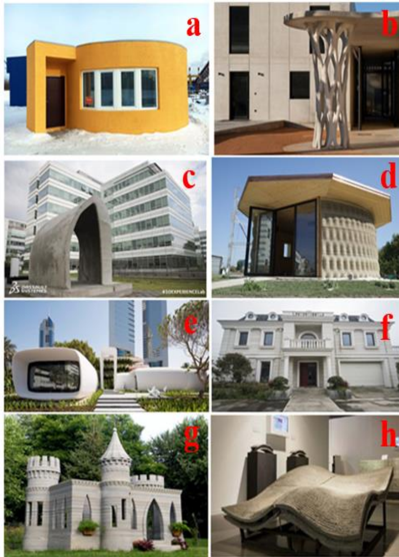
Fig. 18: (a). 3D printed Concrete house by Apis Cor [(Cheniuntai, 2018) Copyrights © Apis Cor 2018], (b). 3D printed pillar in Aix-en-Provence [(XtreeE, 2016) Copyright © 2019, Springer Nature Switzerland AG], (c). 3D printed pavilion in Europe [Copyrights © (XtreeE, 2017)], (d). 3D printed Gaia house using natural materials such as soil and waste from rice production [(Chiusoli, 2016) Copyrights © WASP 2016], (e). 3D-Printed Office Building in Dubai [(Musa et al. , 2018) Copyrights ©Dubai/REUTERS], (f). 3D printed Western-style villa [Copyrights © (Winsun, 2016)], (g). 3D printed Concrete Castle [Copyrights © (Rudenko, 2016)], (h). 3D printed concrete surface [(Costanzi, 2016) Copyright © Loughborough University 2016, UK]
